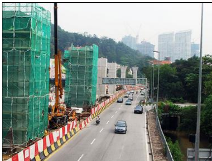
Plate ES-1 Example of the pier constructed at the median of the road for SBK Line
