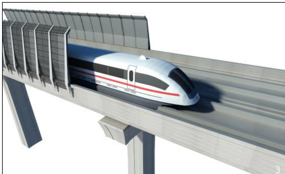
Plate ES-5c Extended height noise barrier with architectural aesthetic screen
