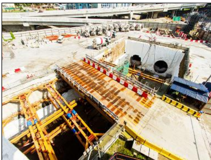
Plate ES-4 Example of the retrieval shaft for SBK Line (Maluri Portal)
